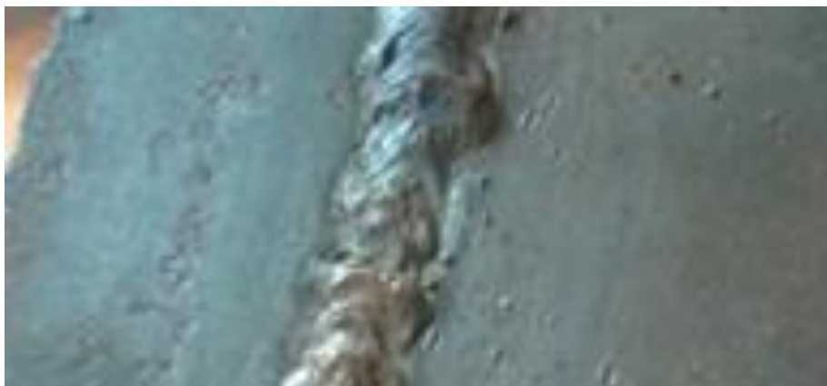
Figure 5.6 - Sample of welded joint
