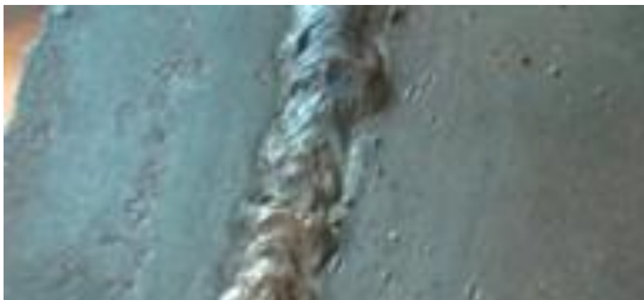
Figure 5.6 - Sample of welded joint
